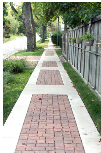
Adding permeable space to concrete, like these blocks of brick pavers, can increase the amount of rainfall that is absorbed by the ground, helping to reduce runoff.
